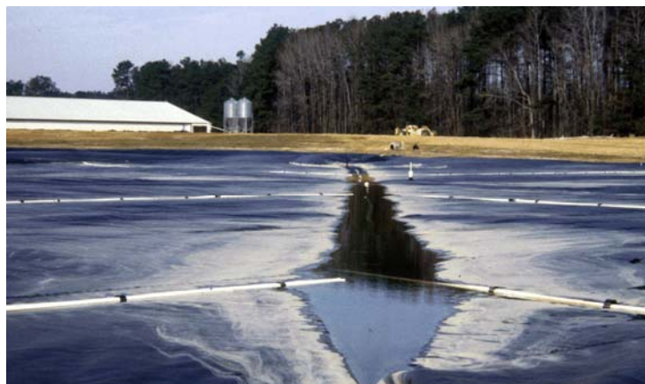
Figure 3-7. Covered Lagoon Reactor (courtesy PSU).
