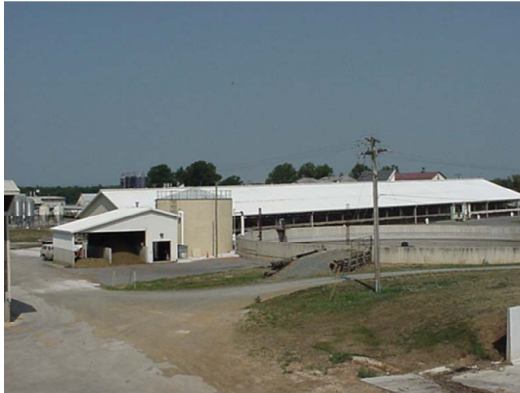
Figure 3-6. Dairy Manure Anaerobic Digestion Facility.
