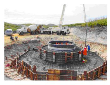
Figure 3-2. Construction of Typical Spread Footing Foundation.
